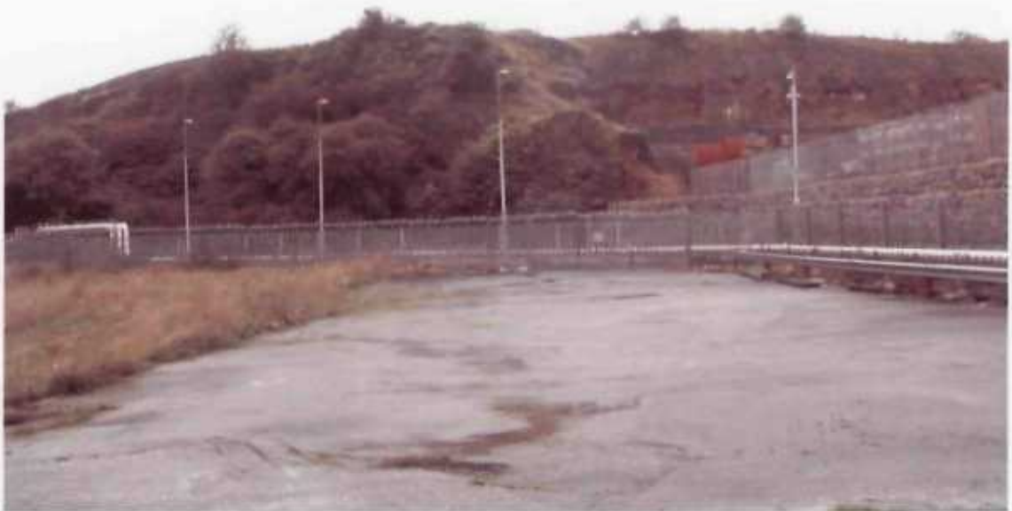
Plate 2: North-west corner of site
